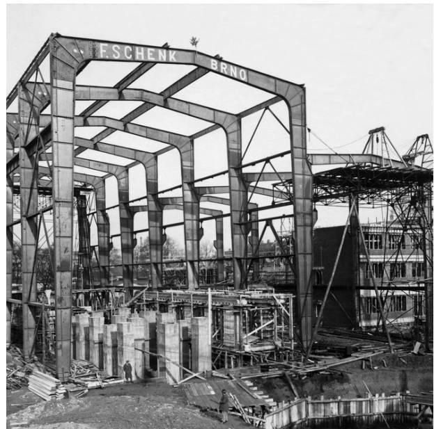
Building of heating plant under construction, 1927-1930
